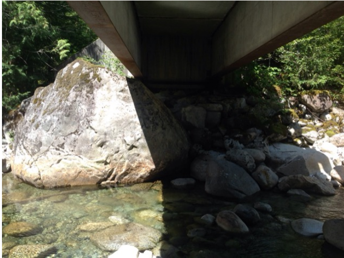
Right Bank Abutment when facing downstream
