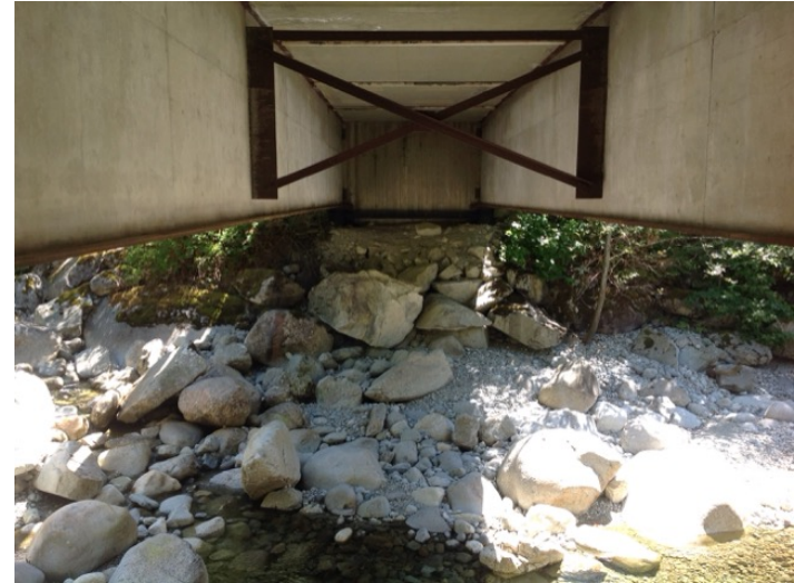
Left Bank Abutment when facing downstream
